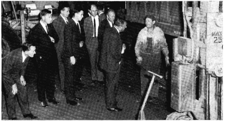
As part of their course, a group from the Australian Administrative Staff College inspected some railway installations last month. They are shown watching operations at the bogie exchange.
