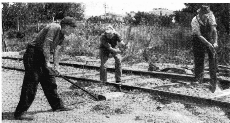
Gang No. 14 replaces sleepers at Welshpool. (From left) Repairers A. Prendergast, A. Humphrey, and Ganger W. Johnson.
