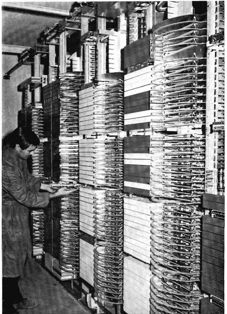
Telephone Technician P. Wells at work in the new Spotswood exchange.
