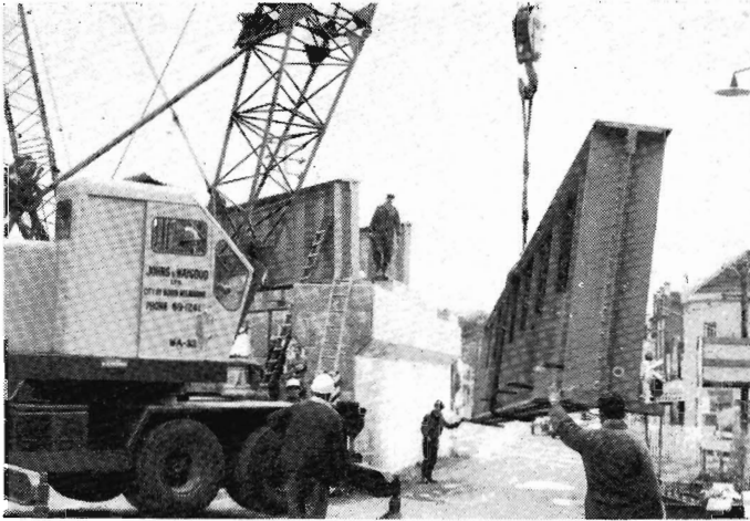
GRADE SEPARATION : Girders are being placed in position over Canterbury Road, to carry the new up track. This $1,600,000 project at Canterbury involves the building of more than half-a-mile of temporary track, a temporary station, an overpass carrying the new track above Canterbury Road, and the construction of a new station about 20 ft. above the site of the old one.
