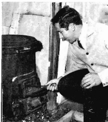
(Below) Mr Brown stokes the boiler.
