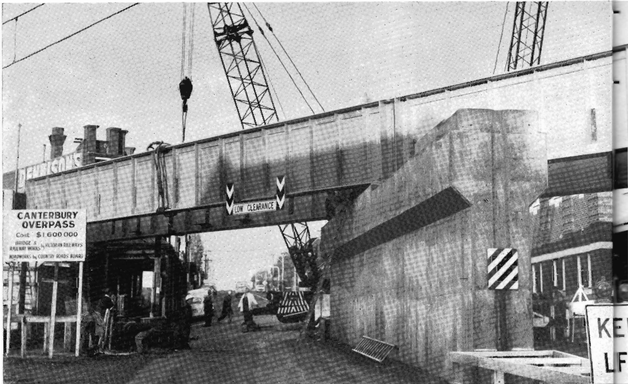
GRADE SEPARATION : Girders are being placed in position over Canterbury Road, to carry the new up track. This $1,600,000 project at Canterbury involves the building of more than half-a-mile of temporary track, a temporary station, an overpass carrying the new track above Canterbury Road, and the construction of a new station about 20 ft. above the site of the old one.
