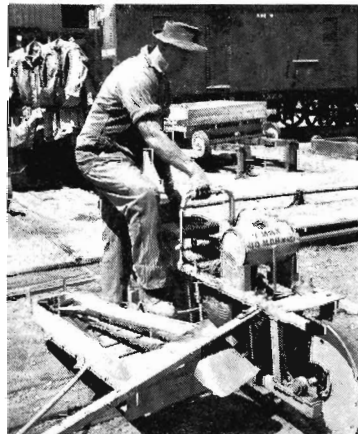
Ganger A. Lacy takes out inspection motor.
