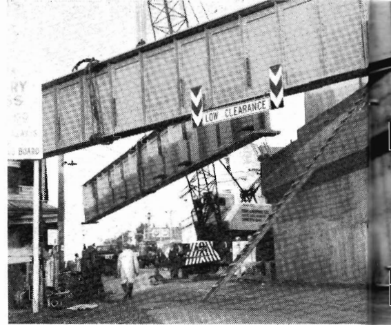
GRADE SEPARATION : Girders are being placed in position over Canterbury Road, to carry the new up track. This $1,600,000 project at Canterbury involves the building of more than half-a-mile of temporary track, a temporary station, an overpass carrying the new track above Canterbury Road, and the construction of a new station about 20 ft. above the site of the old one.
