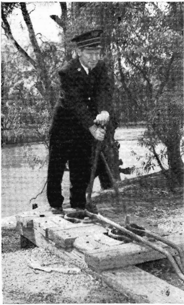
Against a River Murray background, Stationmaster R. McCloskey operates a point lever.
